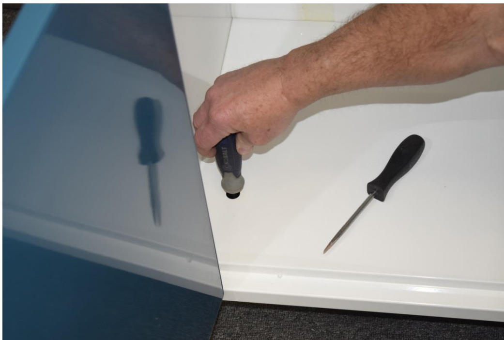
Adjust feet up or down to level cabinets
