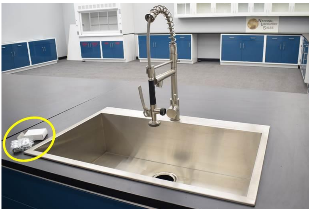
Place the sink and faucet into the hole you cut, and use the provided hardware (circled above) to secure it in place
