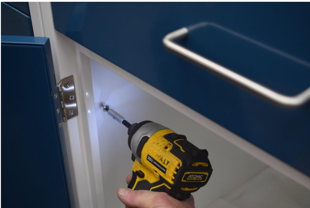
Attach cabinets together using self-tapping screws
