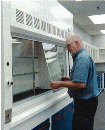
INCLINE AND PUSH INTO THE UPPER GUIDE
