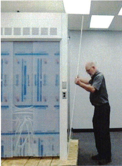
INCLINE AND INSERT PANEL BOTTOM CATCH INTO THE STRUCTURE LOWER LIP
