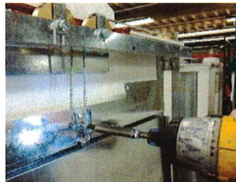
INSERT CLAMP THROUGH BACK AND SECURE WITH 2 SCREWS
