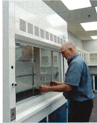
BRING TO VERTICAL AND DROP INTO THE BOTTOM RAIL
