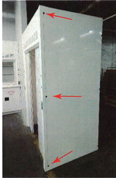
BRING PANEL TO VERTICAL AND LOCATE SCREW HOLES
