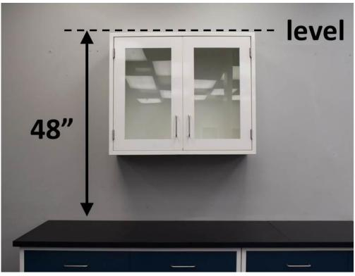
**Hang cabinets on brackets.** Double check that the top of the wall cabinet is level and 48" from the countertop. If it is not level at 48", it is <u>NOT</u> positioned on the bracket correctly.
