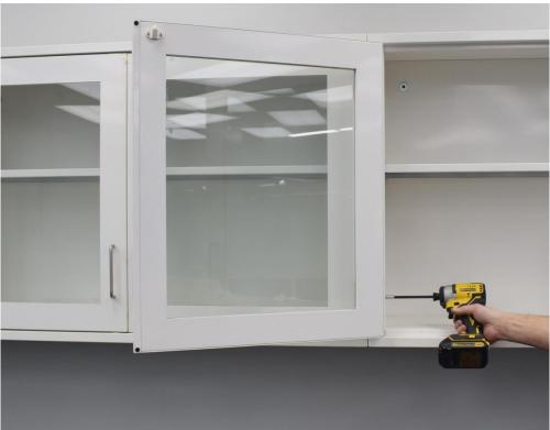
If you have more than one wall cabinet (in a row), screw the units together using short screws located to the front (close to the doors) where you will not come in contact with them.
