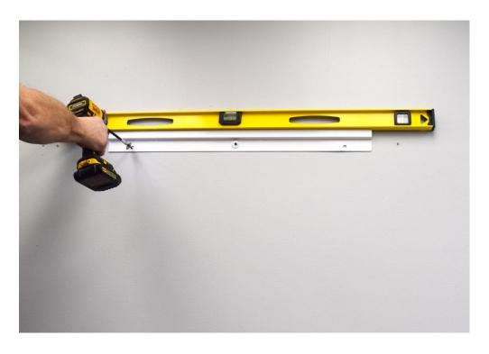
Next, using a level to ensure the bracket is level, finish screwing the bracket to the wall
